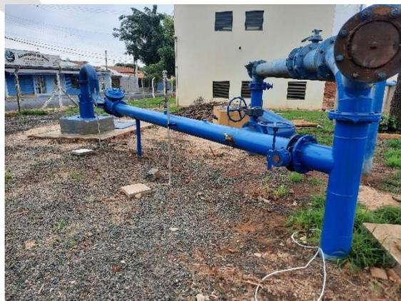
**Figura TEC 3 - Poço Tubular Profundo Iguatemi**
